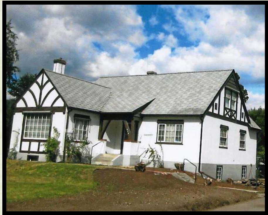
Wasson House on Royal Avenue, March 2014
