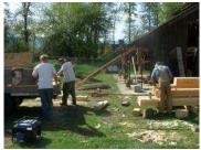
A significant amount of the board and batten ponderosa pine siding is being reattached and repaired. Much of the material had been removed in order to facilitate the moving of the building, pulled off by vandals or fallen off due to disrepair. Where possible original square nails are being reused as well as new square nails to complete the siding repairs.
