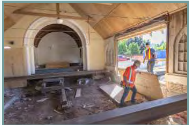
Photo taken by Gary Nylander: Albert Blackwell left and Justin Hunt with Blackwell Building movers take down a piece of plywood that covered a section of the wall in preparation for the building's move.
