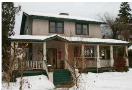
Arthur Dawson Residence, 368 Cadder Avenue Courtesy: Kelowna Heritage Register
