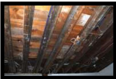
When the kitchen ceiling was removed, a four-inch thick concrete slab was revealed, installed no doubt, over a hundred years ago to keep the original cast iron tub from crashing through the floor boards into the kitchen below.
