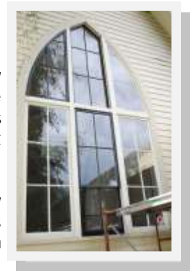
East Window Conservation Process
