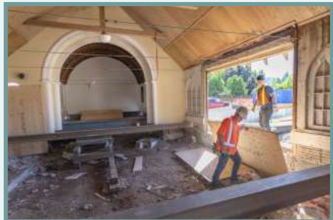
Photo taken by Gary Nylander: Albert Blackwell left and Justin Hunt with Blackwell Building movers take down a piece of plywood that covered a section of the wall in preparation for the building's move.
